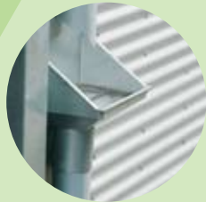
Downspout filters protect the home by preventing gutters from blocking and flooding of eaves. They also reduce a potential fire hazard.
